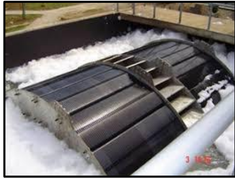
Gambar 51. Rotating Biological Contactor (RBC)
